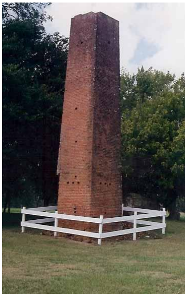
Bynum Chimney Stack
